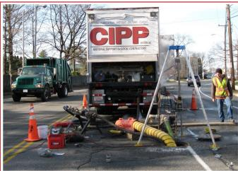
Most of the preparation work for CIPP lining can be done during a normal work day. Sometimes when the liner size is larger the resin requires more time to cure. During this cure time the machines that are running is the bypass pump and the boilers. Once the line is cured the pipe is cut and the services are reinstated.
