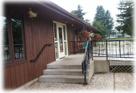
Clubhouse entrance from the parking lot
