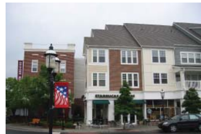
Window and door openings
