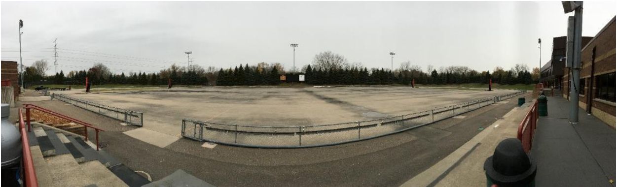
Wide angle picture of the refrigerated ice slab.
