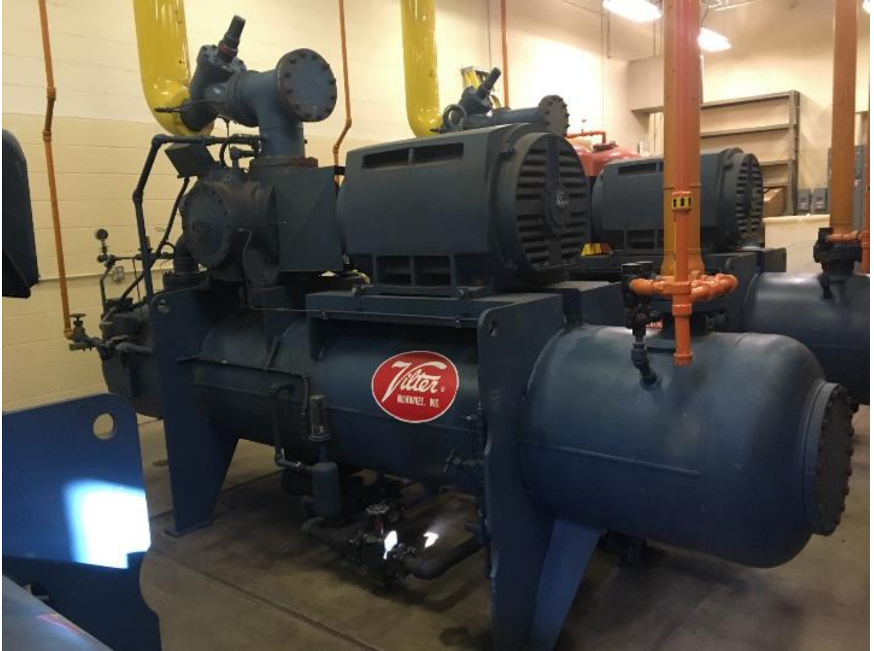
Twenty-five-year-old Vilter Screw Compressors
