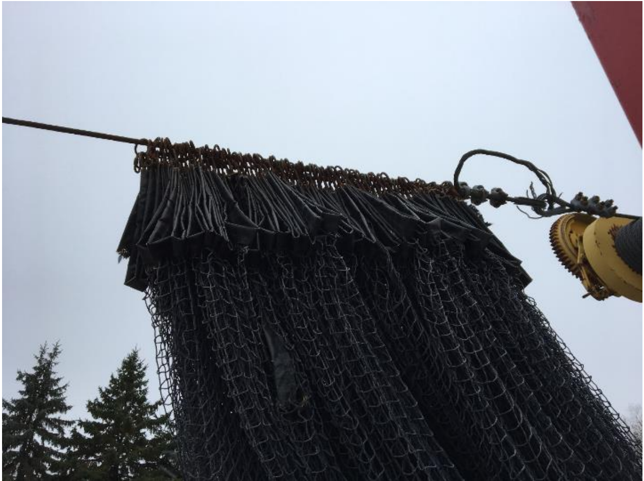
Worn and weathered netting between speed skating loop and center hockey rinks
