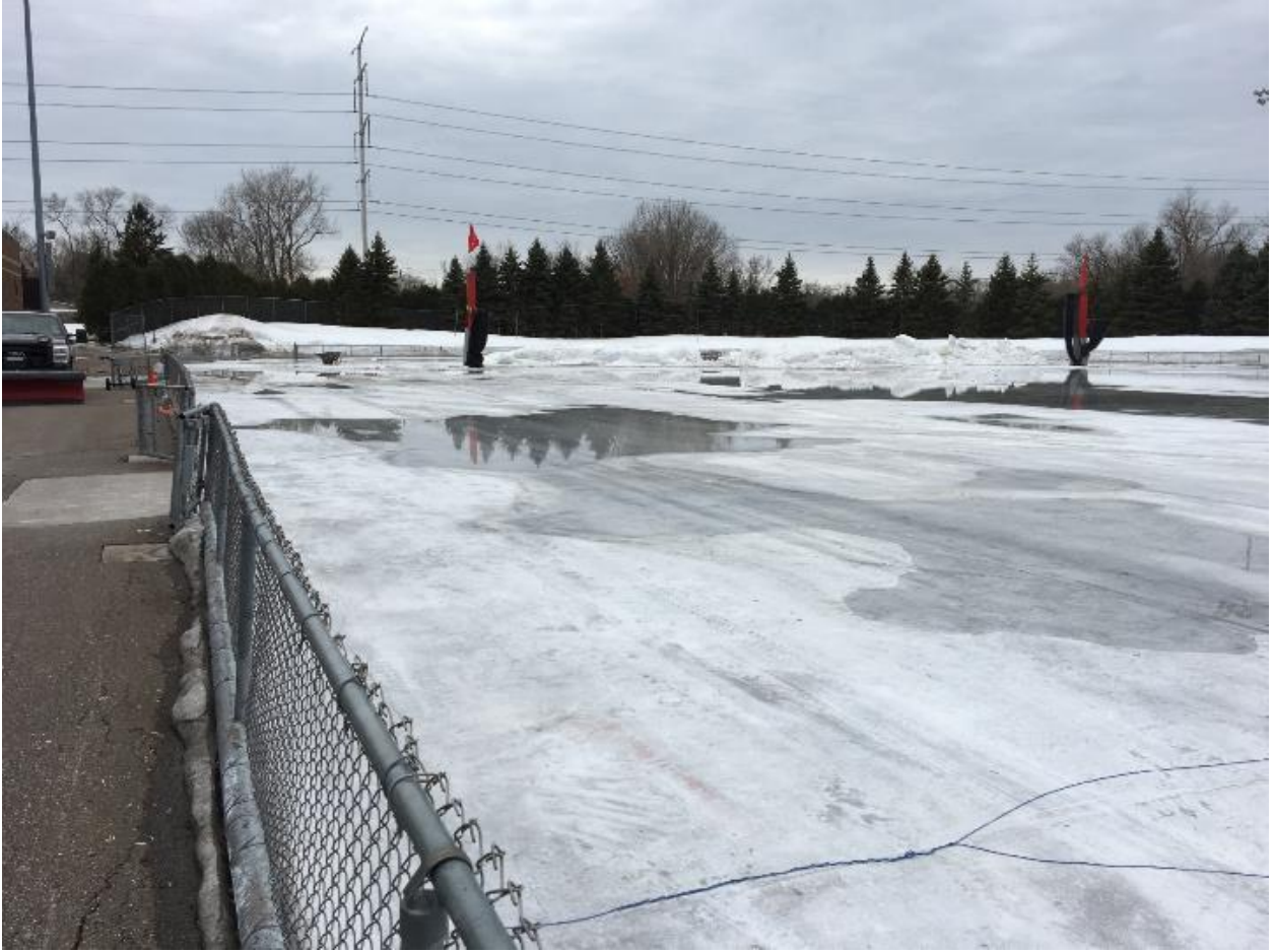
Pool ice slab drainage due to winter frost heave
