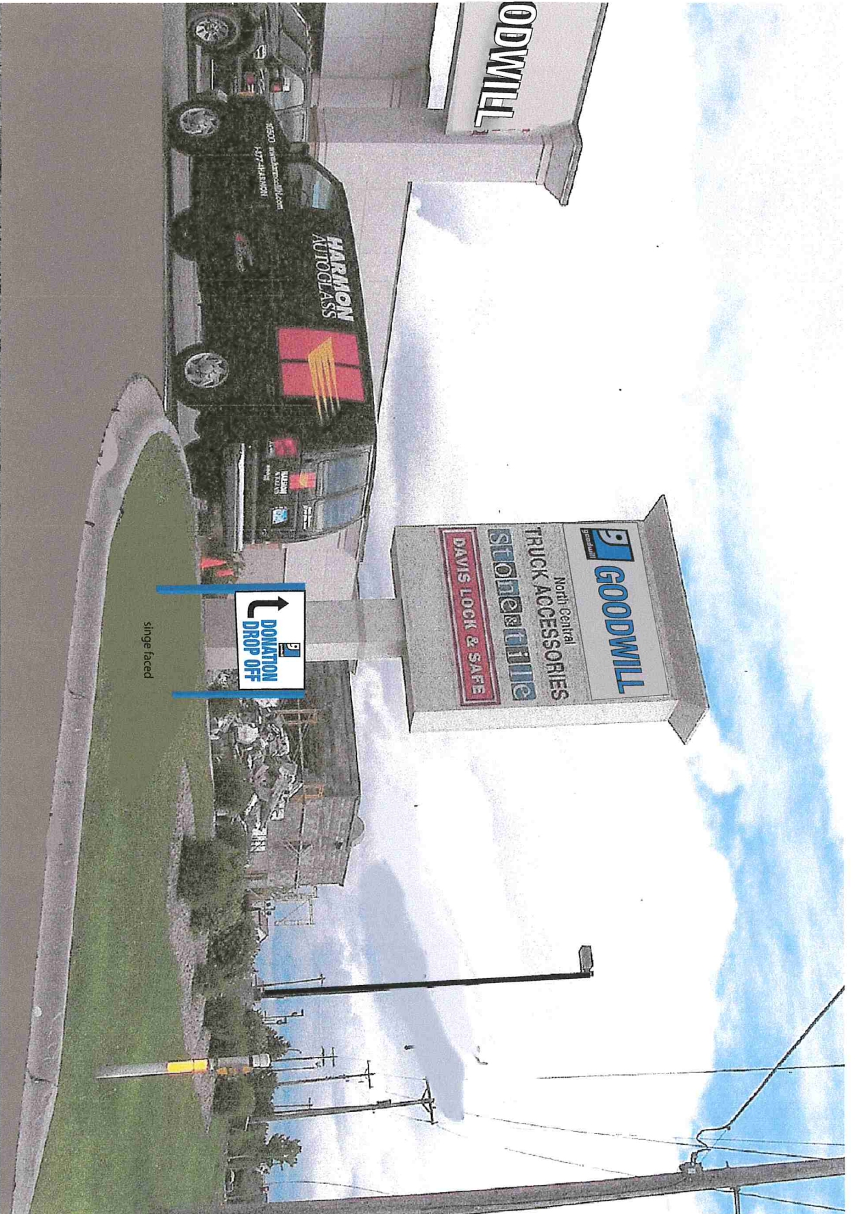
Goodwill -Roseville Post & panel S/F 18" X 30" with 2"x 2" alum sq. tube - non illuminated
