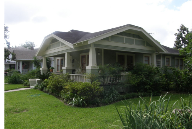
Bungalow w/wrap-around porch
